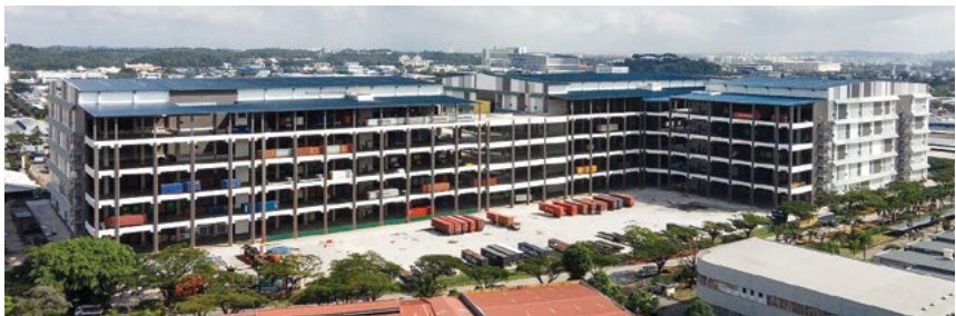
Solar PV will be installed on the roof of AA Reit's largest logistics and warehouse property in Singapore, at 20 Gul Way.
