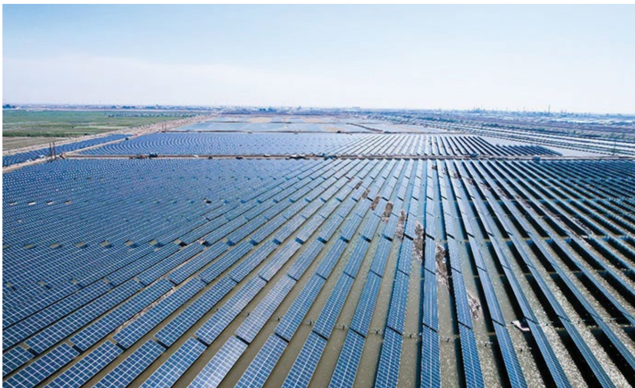
Trina Solar's Vertex 670 W modules and N-type Vertex 690 W modules have been installed in a 70 MW fishery photovoltaic project, in China.
