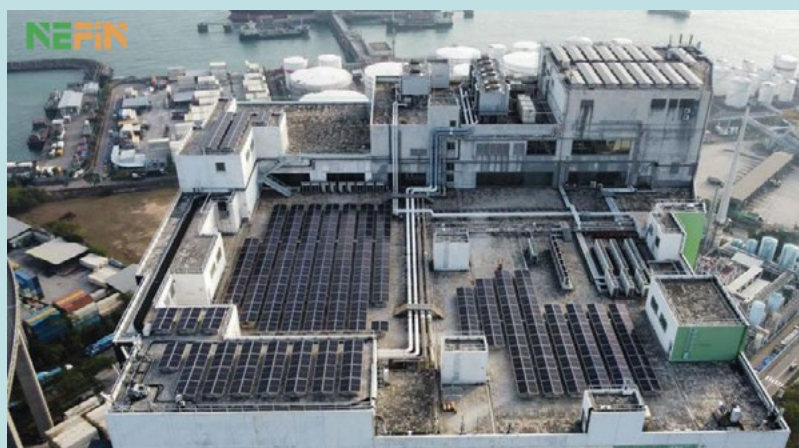
An aerial view of a high-rise rooftop solar project, based on a customised design and the adoption of materials that can withstand strong winds.
