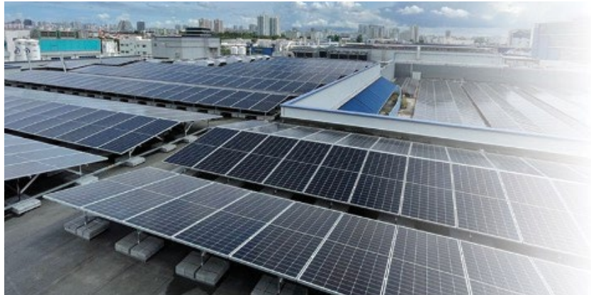
UTAC's rooftop installation will generate over 1,000,000 kWh of green energy annually.
